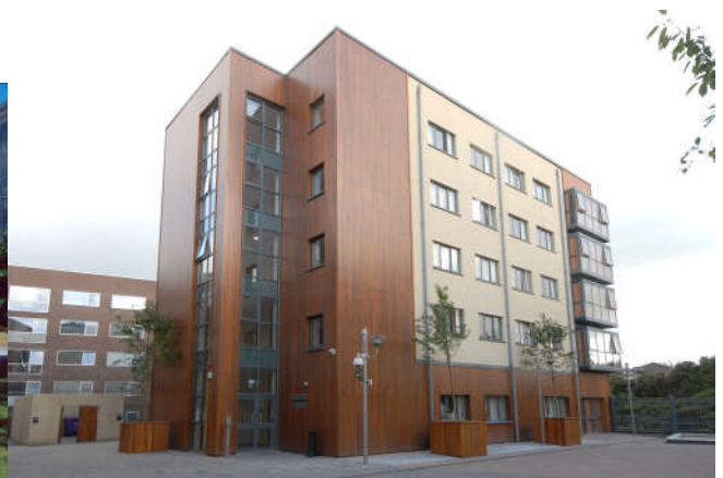
University Hall Apartments Exterior View
